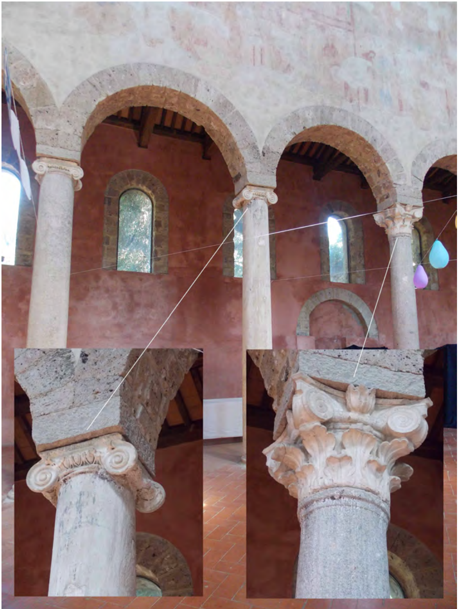
Fig. 1: S. Pietro ad Montes-inside the church. Zoom on the different reused capitals and columns.
