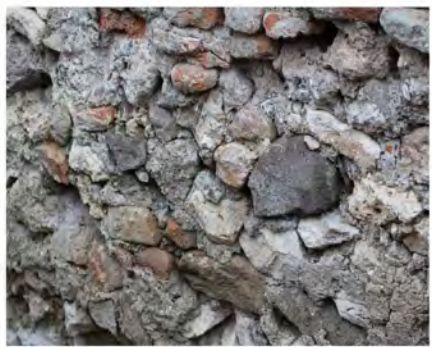
Fig. 5. The Sanctuary of “Maria Santissima ad Rotam Montium” in Leporano: The underground environment buried under Roman concrete (opus incertum) (n. 1), concrete flooring and structural materials (n° 2-3) incorporated into the lower walls of the Sanctuary (© M. DI NIOLA).
