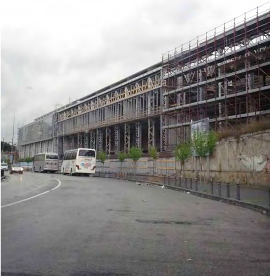
Figure 3: the façade during construction.
