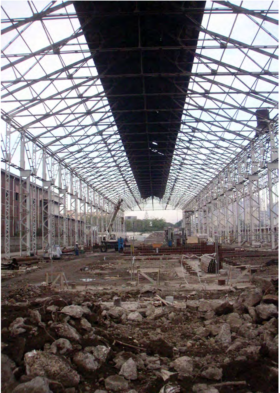
Figure 4: the steel skeleton of the old factory.
