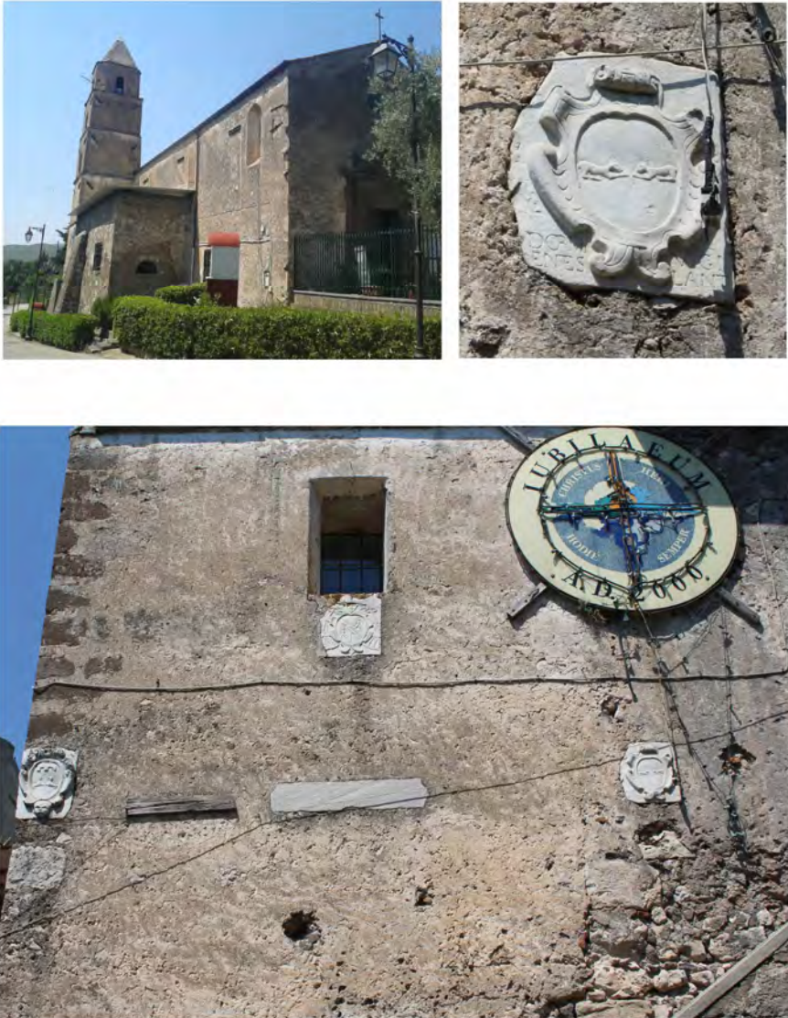
Fig. 4. The Sanctuary of "Maria Santissima ad Rotam Montium" in Leporano. The southern side of the building: the bell tower (n. 1), details of the coat-of-arms-symbol of the community of Leporano (n. 2) and masonry walls (n. 3) portraying incorporated coats-of-arms and inscriptions (© M. DI NIOLA).
