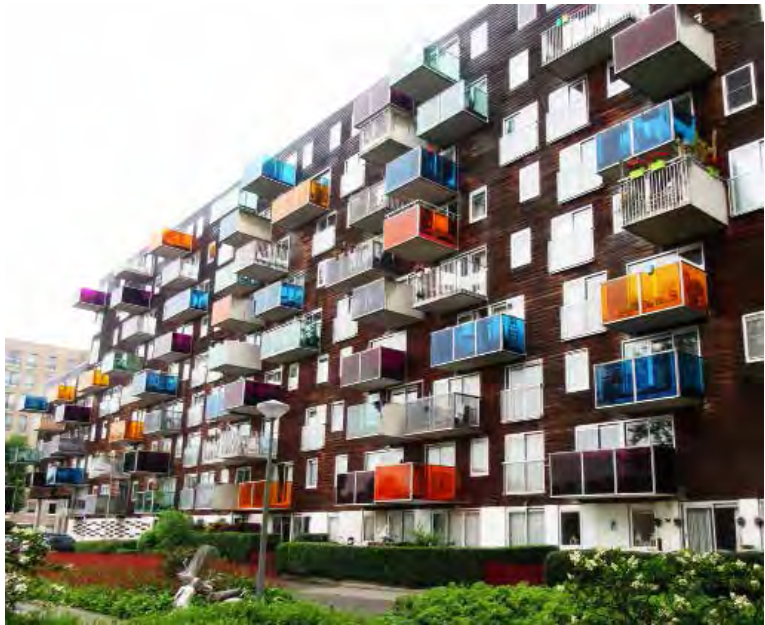
Amsterdam, project Wozoco MVRDV photo: Alessandro Ciambone, site visit August 2017
