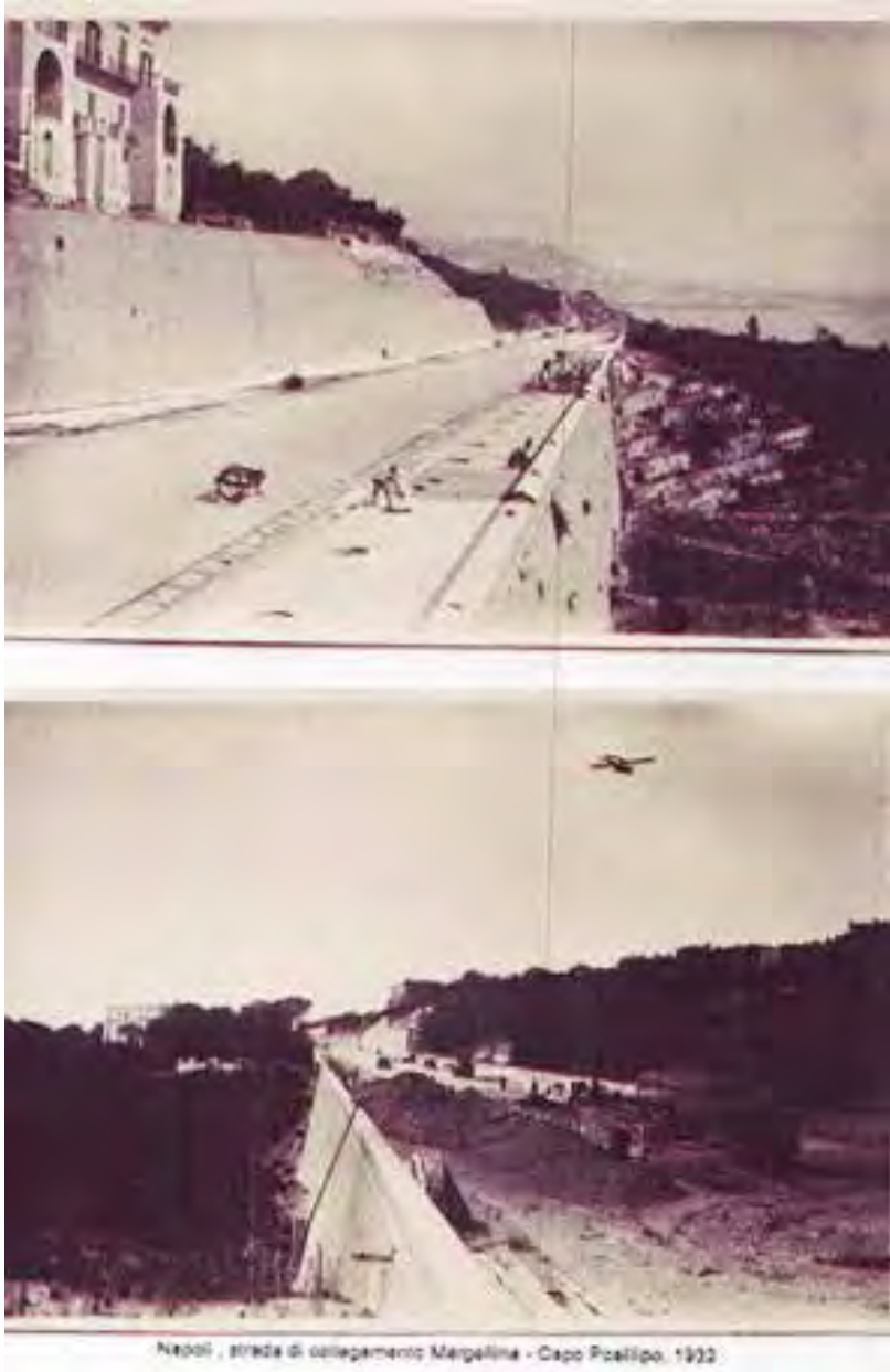
Napoli, via Panoramica (today, renamed via Petrarca) under construction, in 1932 pictures.
